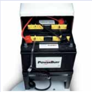
Smart Watering System
